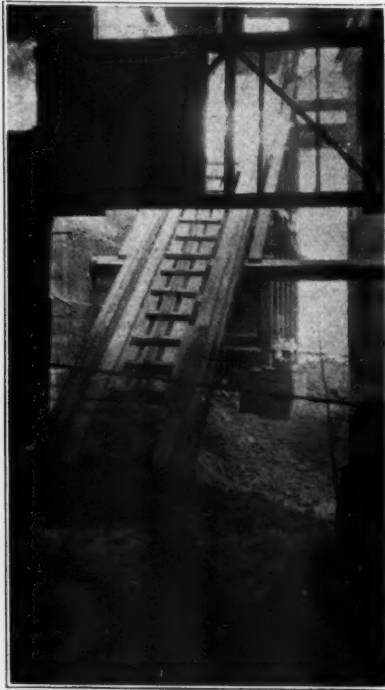
Hoist Taking Waste From Kilns
